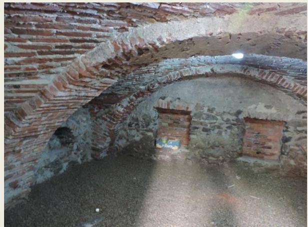
paid special attention to maintain the original, arched form of the roof. The attic is now clear and transparent, if needed, it can easily be transformed into an exhibition-room.
